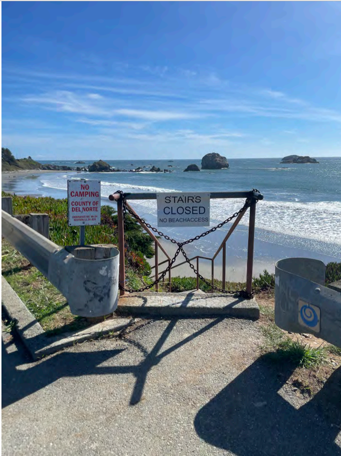
Photo 4. Closure signage at the entrance to the Surfer Stairs restricting public access due to deteriorated stairway conditions.
